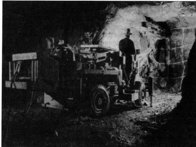
FIGURE 1.6 Small size drill jumbo, Dome mine, Canada
