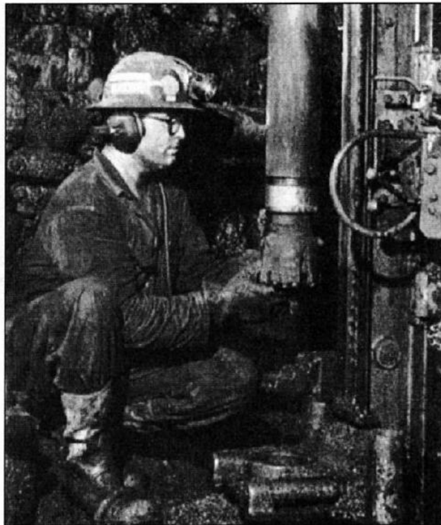
FIGURE 1.15 ITH drilling, 165 mm blast holes, INCO, Canada
